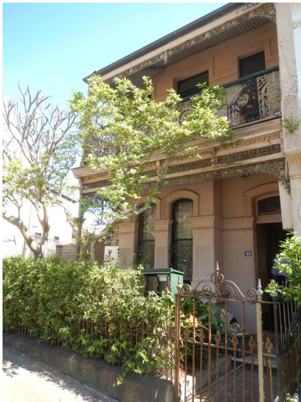
Figure 2. Front façade of 48 Duxford Street, Paddington
